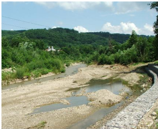
Figure 6 Works to strengthen the banks in the middle sector
