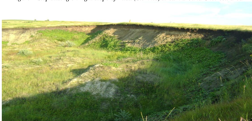
Figure 5 Cornice detachment of 'pit' sliding near town Răduiești on right slope of Stemnic
