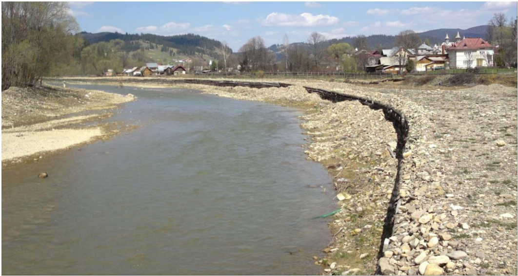
Figure 4: Crib wall bank protection on Moldovita river in bend zone
