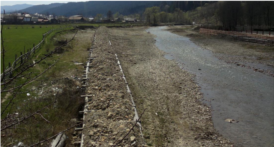
Figure 5: Crib wall bank filling with river ballast
