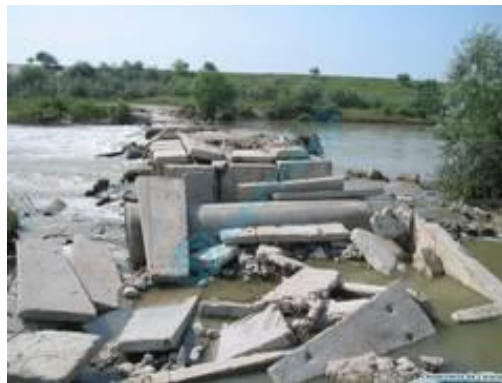
Figure 1: Crossing of the Arges River at Budesti
